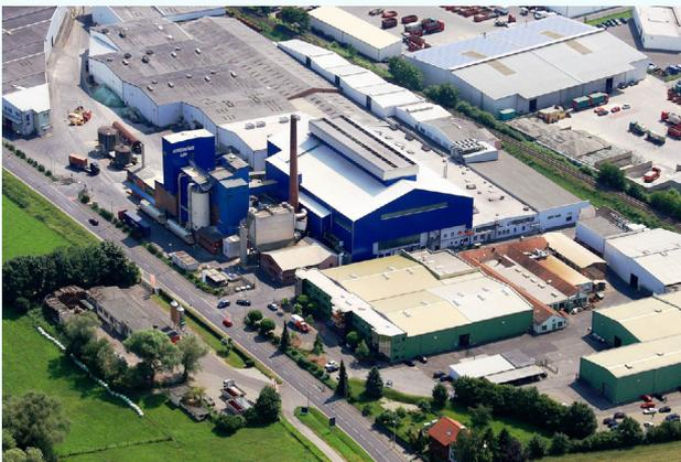
At the Lohr location, Gerresheimer produces more than one billion glass containers for the pharmaceutical and food industry every year with two melting furnaces for clear and brown glass. By using this innovative furnace technology in conjunction with green energy for glass melting, we will significantly reduce CO<sub>2</sub> emissions from production by around 25,000 tons per year.
