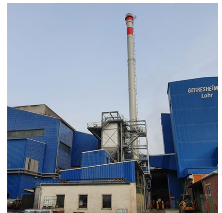
Exterior view of the Lohr plant with new chimney and exhaust gas filter
